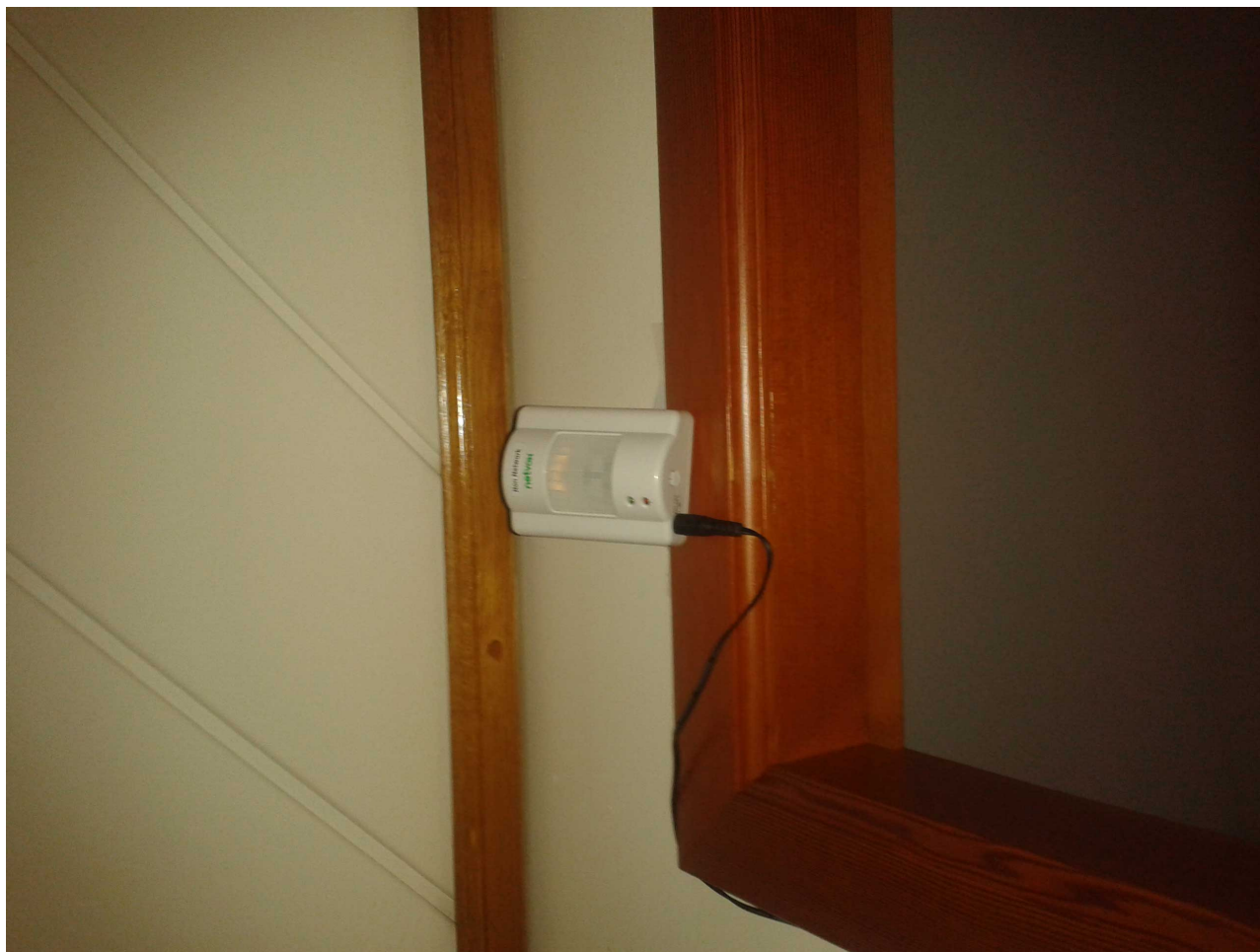
Figure 33 Motion sensor placement
